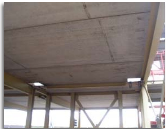
Example of pod opes on Flood Super Wideslab with trimmer beams eliminated.
