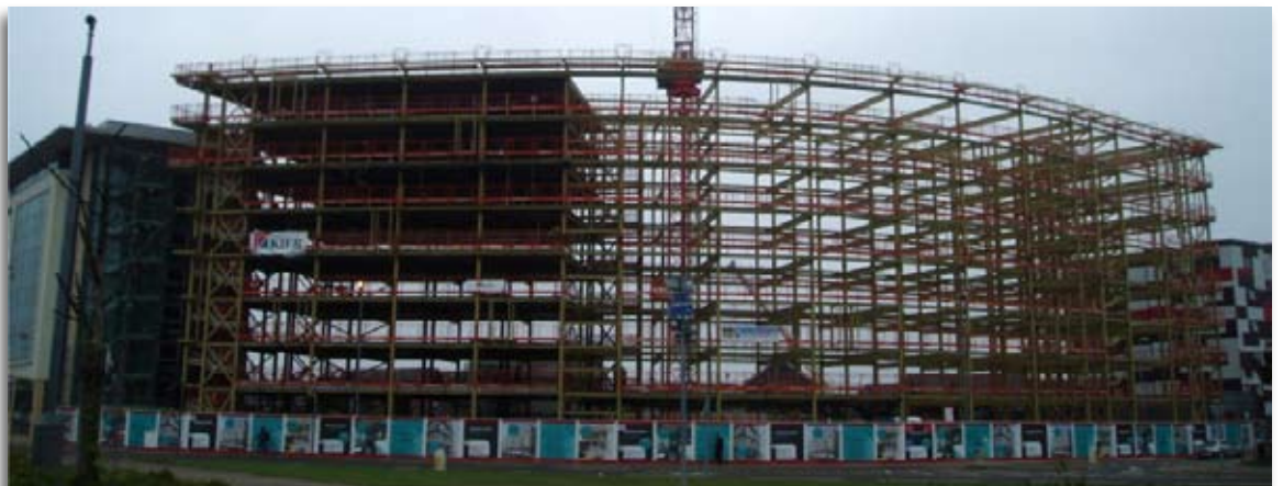
Erection of 2.4m wide Super Wideslab with tower crane.
