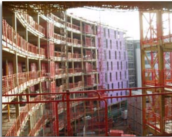
Building profile that required precast flooring units to suit.
