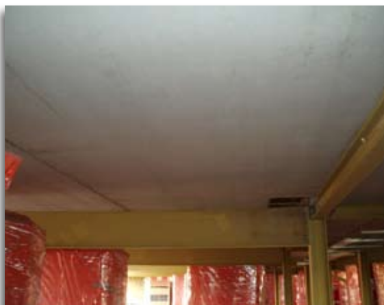
Example of Flood Precast Super Wideslab soffits PRIOR to painting.
