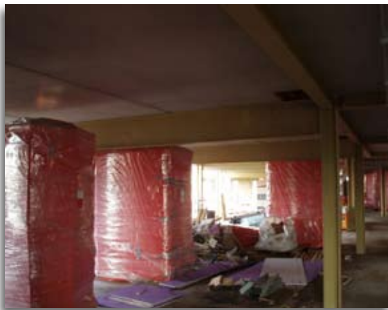
Example of pod opes on Flood Super Wideslab with trimmer beams eliminated.
